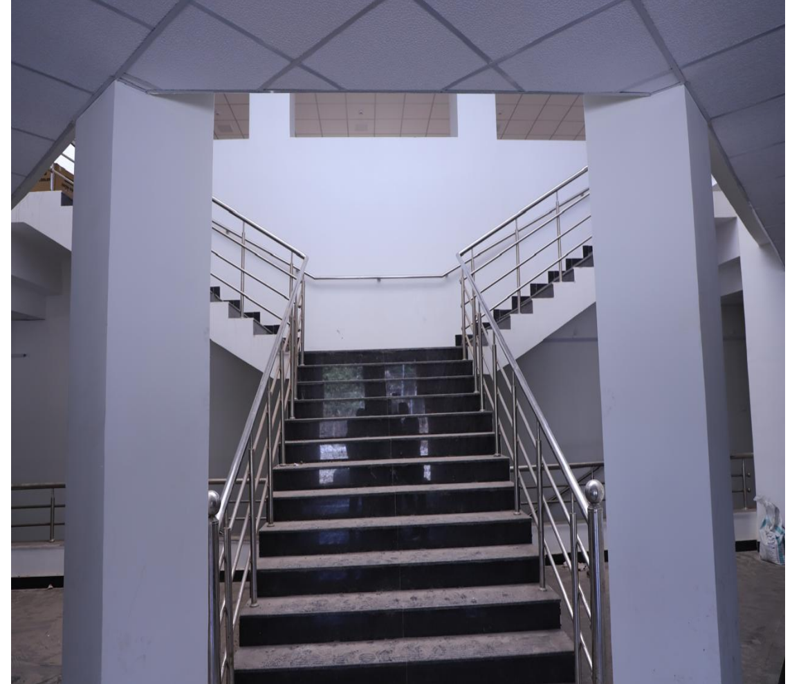
Main Entrance Staircase
