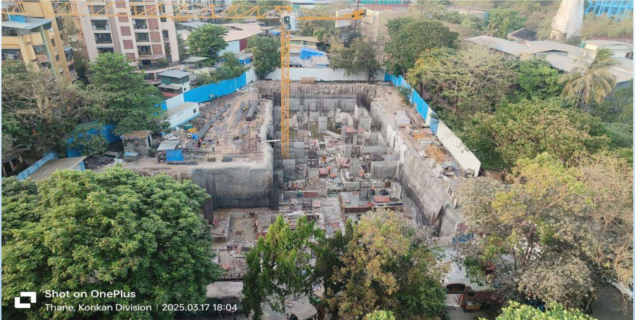
Nursing Training centre and Hostel Building Basement
